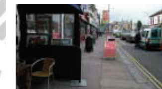
Poor quality street level obstructions and pavements on London Road
